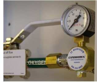
Shown above single port E Z Backfeed™ fitting with Gauge & DISS gas specific demand valve
