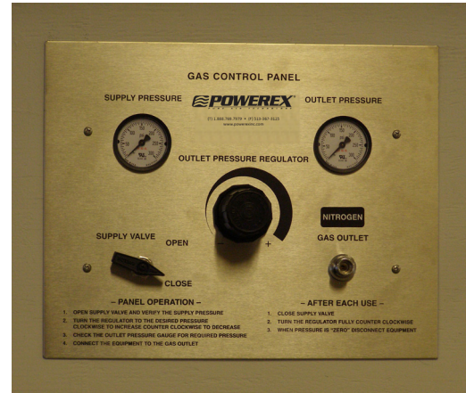
PX-NP100 – Nitrogen Gas Control Panel
